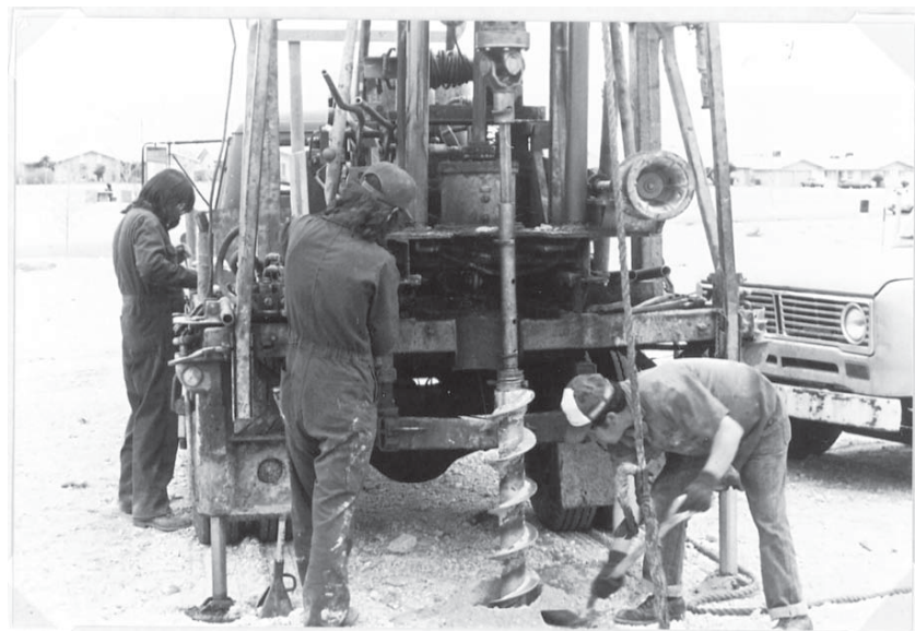
Figure 3: Drilling with continuous flight augers
