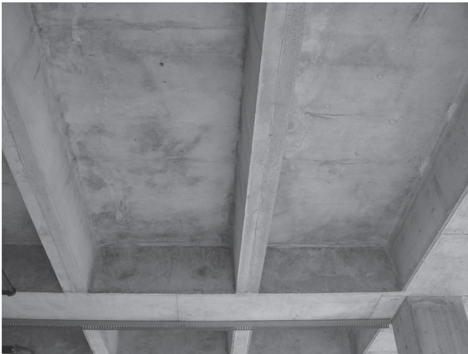
Figure 12.3-3: Skip joist system showing wide spacing between ribs.
