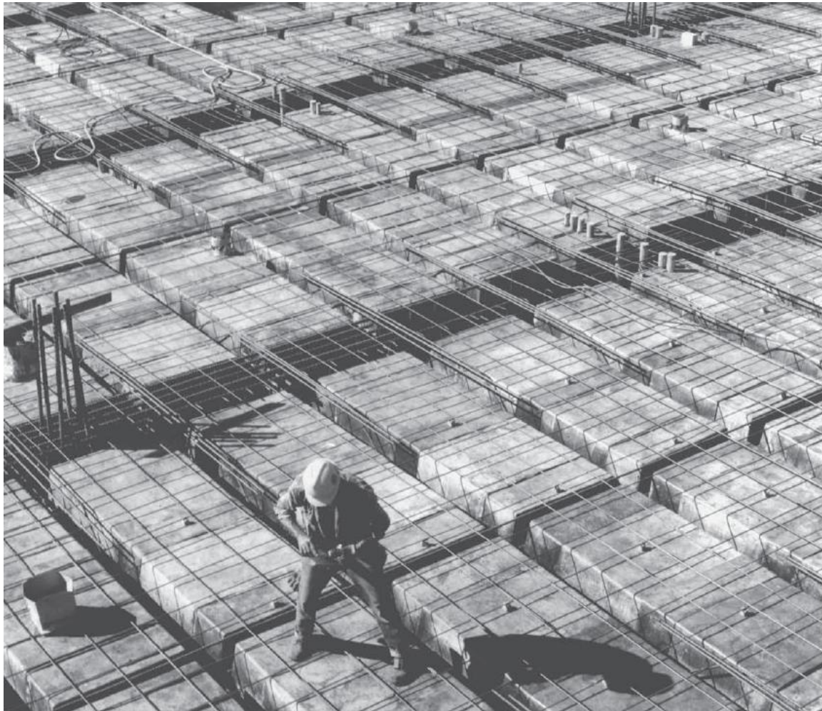
Figure 12.3-1: Steel forms for one-way joist floor.
