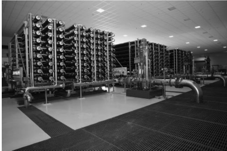
Figure 17-2 Typical reverse osmosis facility.
